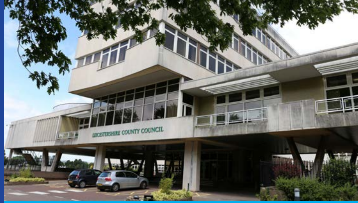
Leicestershire County Council building
